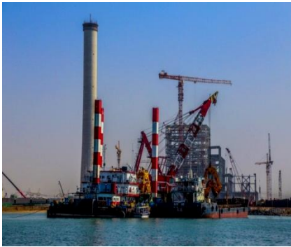
Hub Coal Power Plant
