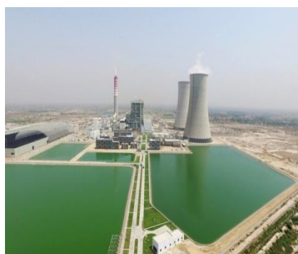
Sahiwal Coal Power Plant
