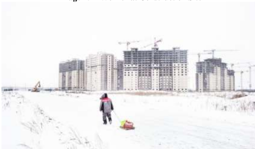
Image 2: A Worker at Construction Site
